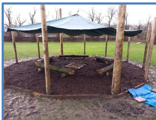
The new outdoor classroom being built
